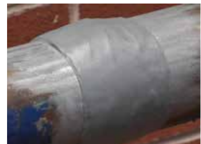
Leak repair completed
