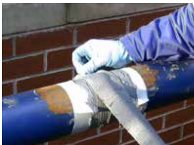
Belzona 9341 applied to perform a wrap repair
