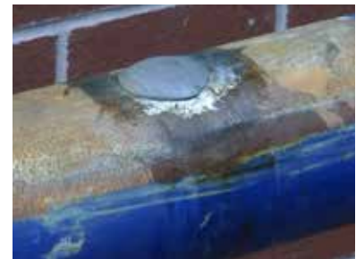
Belzona 9611 stops the leak
